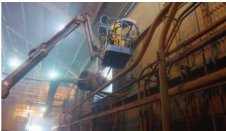
FIGURE 2. As part of the dust-sampling and hazard-assessment plan, it is important to collect representative samples of fine powdered materials that may be present in the facility. Keep in mind that fine particles are often found in elevated locations, such as ceilings, walls and ledges
